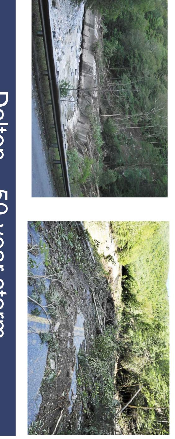
Right, below: Rt. 2 road collapse and landslide along Cold River in Florida & Charlemont
