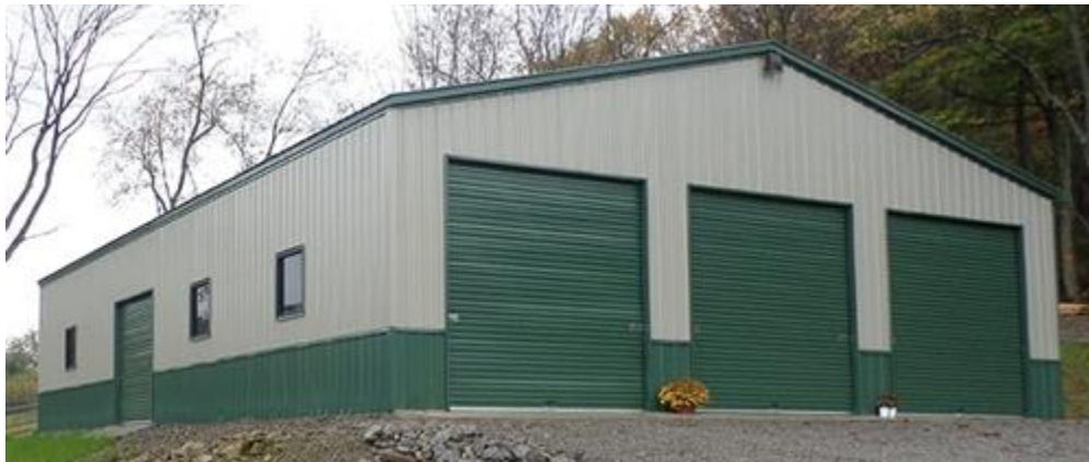
Typical pre-engineered building (Final design will vary from photo)
