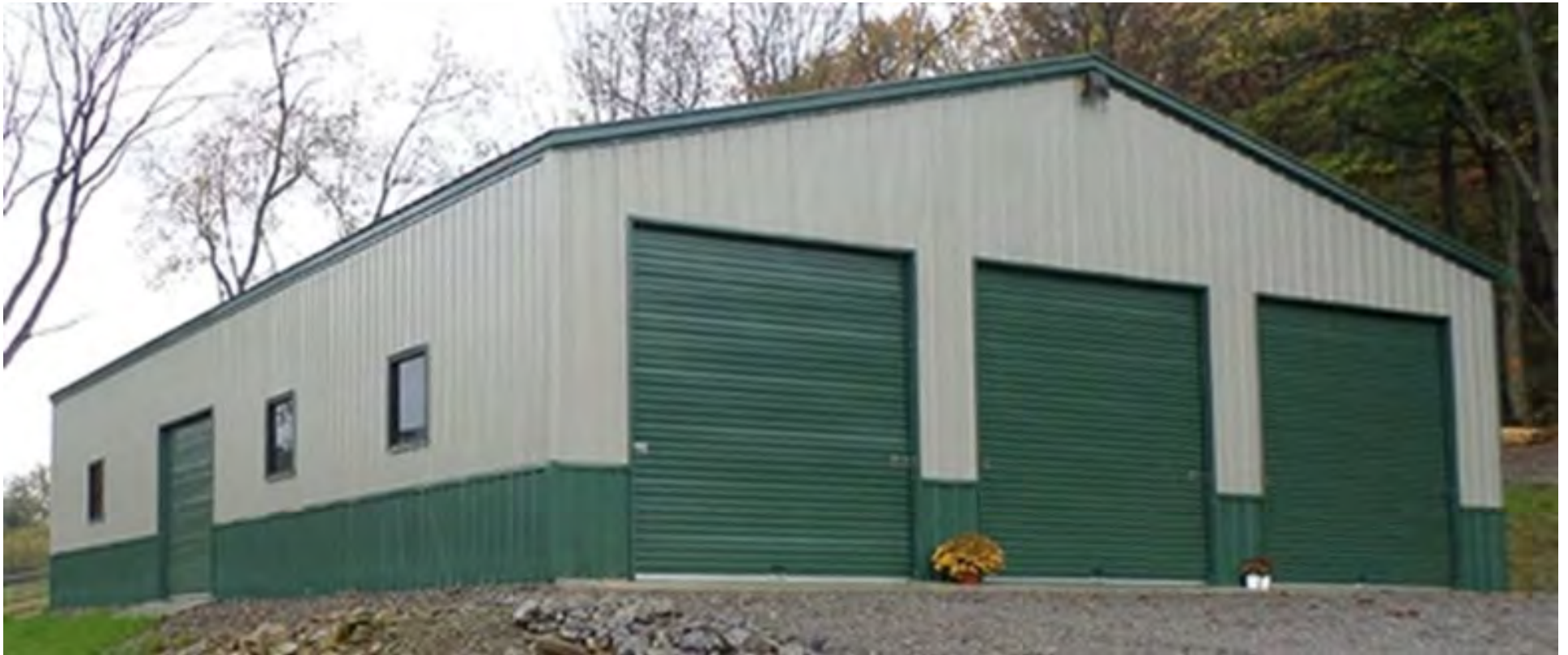
Typical Metal Building Photo
