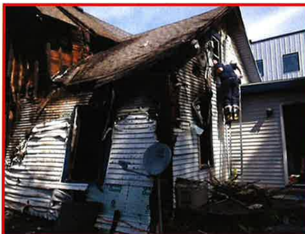
Explosion and resulting fire caused by extracting hash oil using butane.
