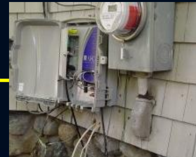
Subscriber's Optical Network Terminal (ONT)
