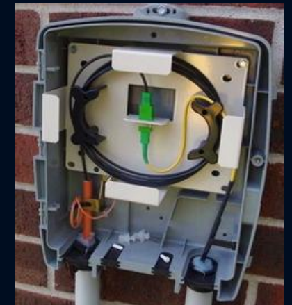
ONT housing w/o ONT installed
