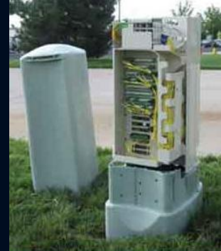
Fiber Access Terminal (FAT) or Pedestal
