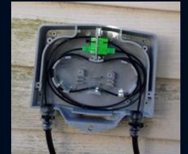
Fiber Transition Terminal (FTT)
